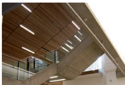
Pre-fab panels showing vertical shadow gap
