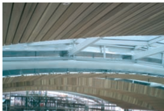
Concealed fixing details mean the ceiling has clean, uninterrupted lines, as well as providing a durable solution.
