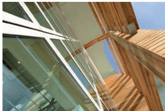
Timber clad Glu-lams & fixings to cross-beams
