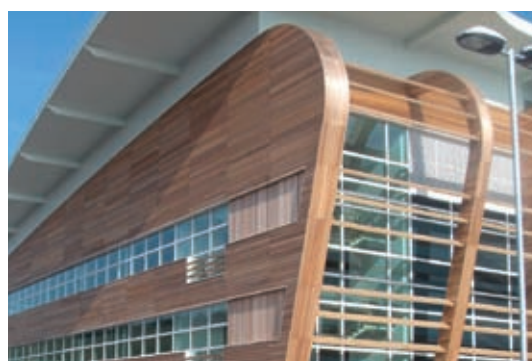
West elevation with secret-fixing horizontal panels and aluminium feature trims
